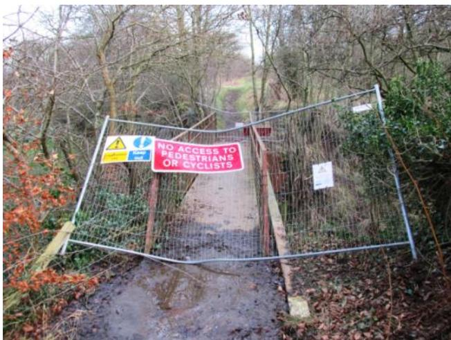
The bridge over the Garrion burn, between Waterloo and Law has been closed for Public safety (the 'I' beams are corroded, and abutments are scour damaged).
