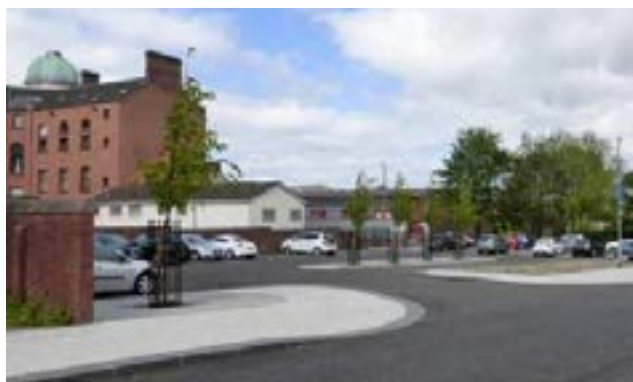
Refurbished car park Coursington Road / Dalziel Street
