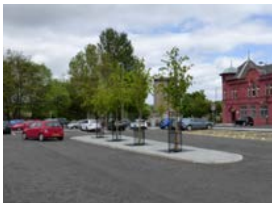
Refurbished car park Coursington Road / Dalziel Street
