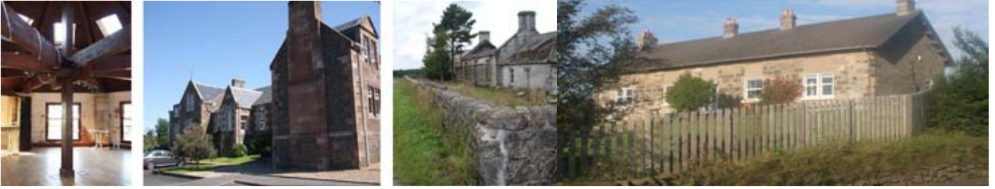
Restored interior Former school converted to houses Conversion possibilities Former School converted to a house
