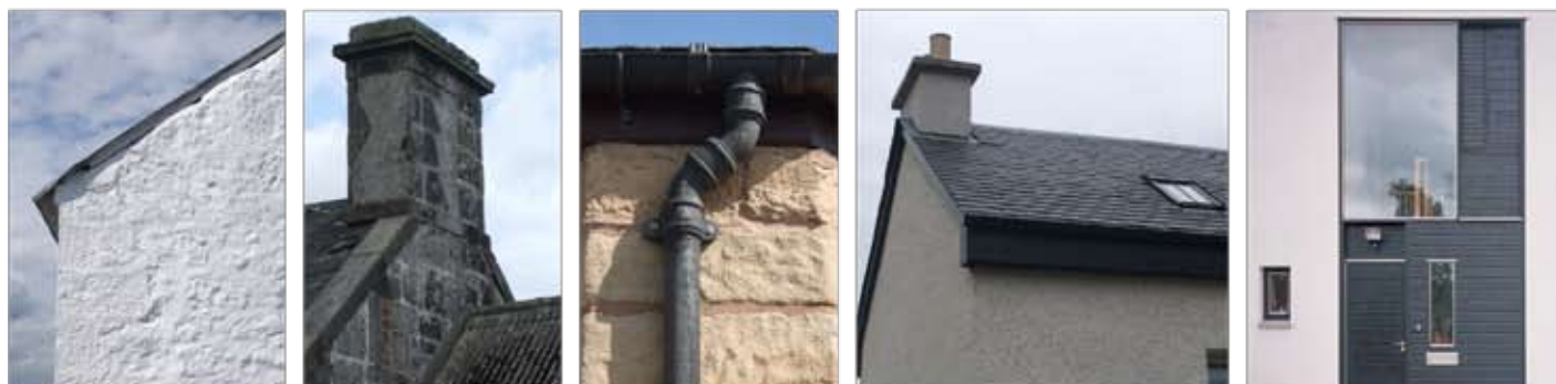
Retaining and reflecting traditional details and materials - from white painted roughcast render, semi-dressed local stone; metal gutters & downpipes; - can be carried through to modern textured rendered walls with slate roof, or smooth render with timber details.
