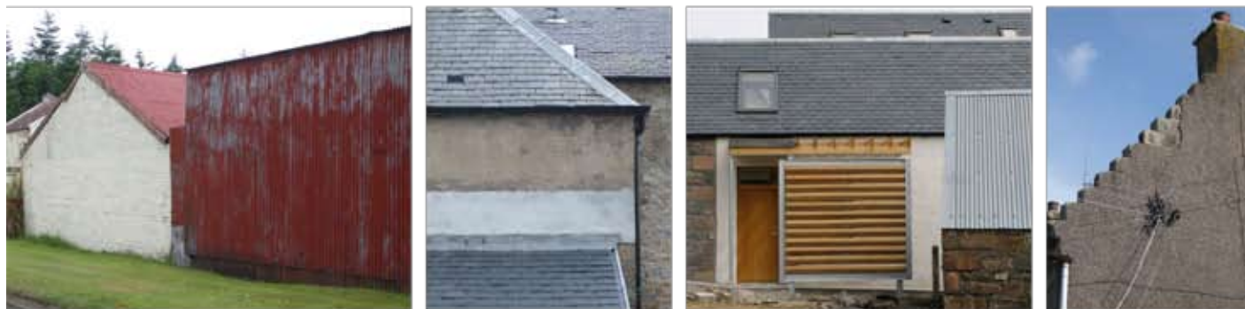
Reflecting diverse local materials can help development fit in - whether painted metal corrugated sheeting, slate roof with lead flashings, to timber doors, windows and screens and crow-stepped gables
