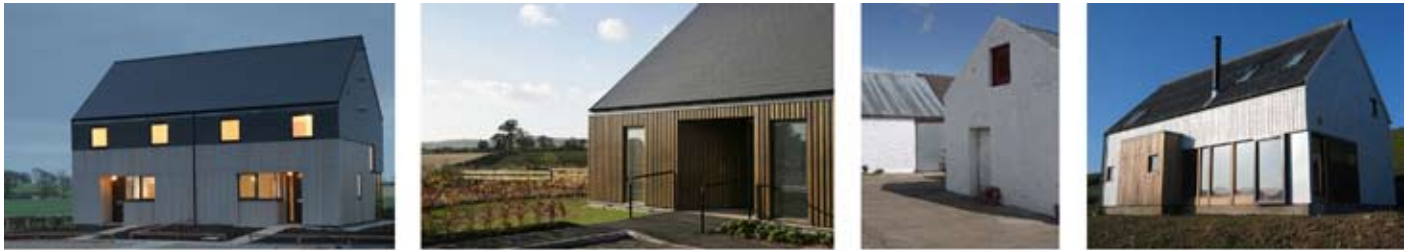
Simple traditional forms can echo the agricultural character. There is usually a need to balance proportions and extent of openings.
