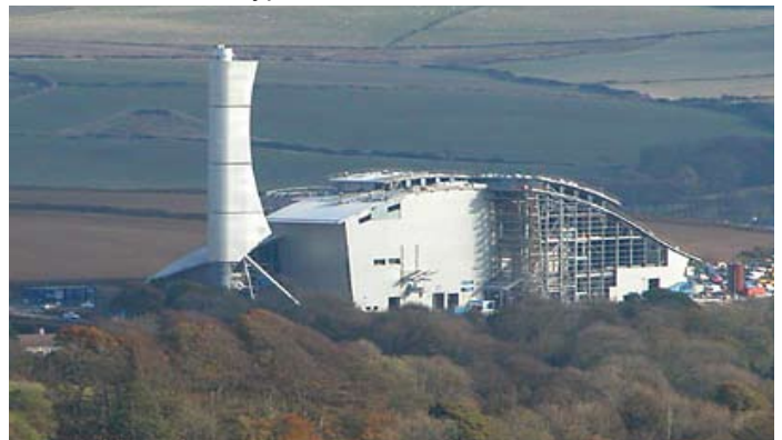
The Isle of Man government's new award winning Energy-from-Waste (EfW) facility (above right and below) - not trying to hide, but creating a landmark with a sail shaped stack and curved main structure to fit in with the surrounding hills. Includes 16-day storage capacity; reuse of rainwater; and on-line emission monitoring data.
