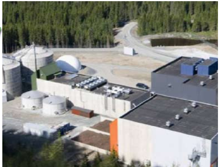
Anaerobic Digestion Plant
