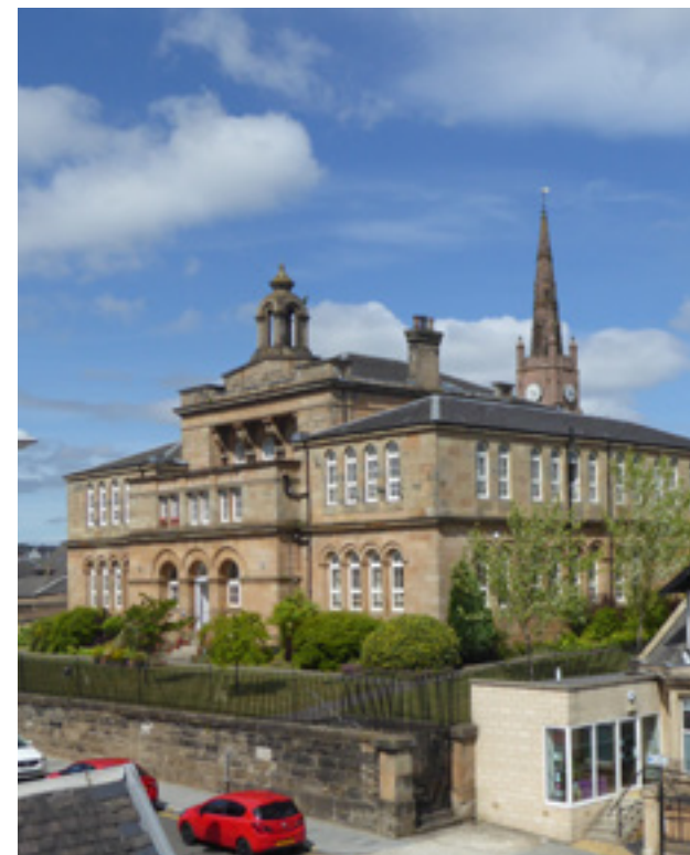
Former Gartsherrie Academy, Coatbridge
