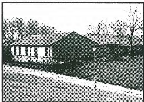
Special needs housing under construction at Seafar
