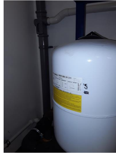
Booster Pump Expansion Vessel
