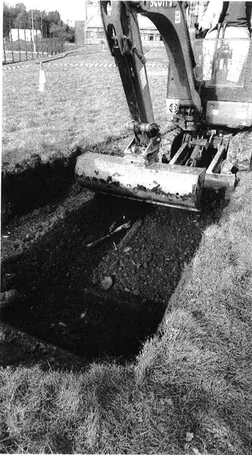
Machine excavation in progress
