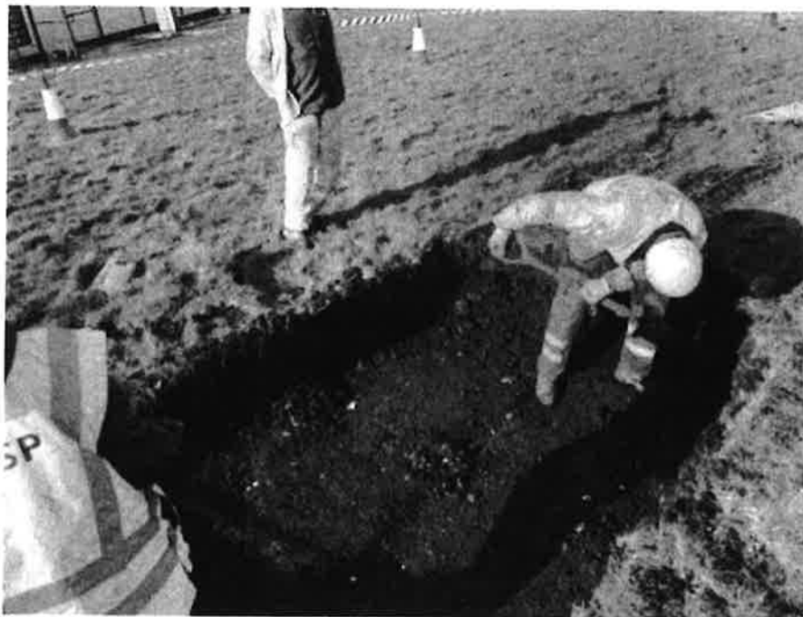
Hand excavation of topsoil in remedial area surrounding HP10.
