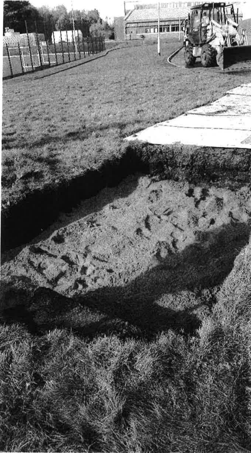
Backfill with sand subbase
