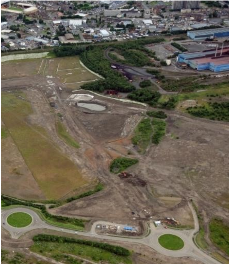
Aerial view southwest from existing roundabout at Ravenscraig Regional Sports Facility across Ravenscraig and the line of the proposed development to Motherwell.
