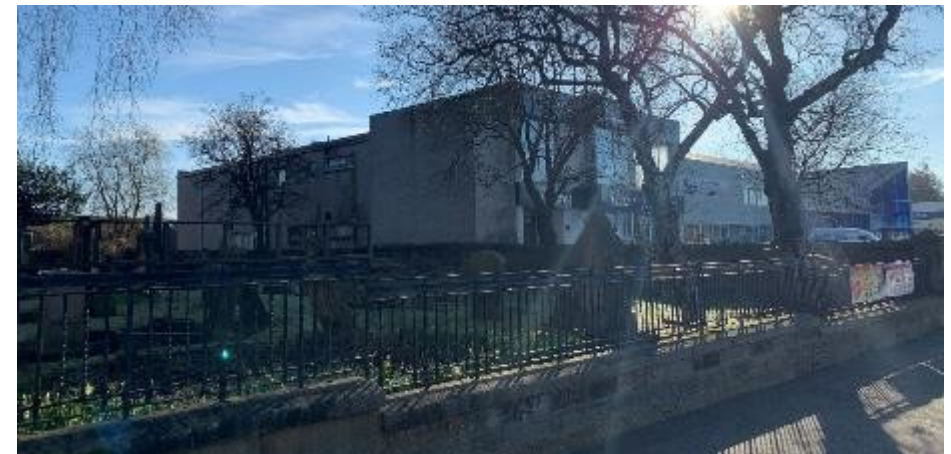
View looking from Windmillhill Street of existing commercial premises
