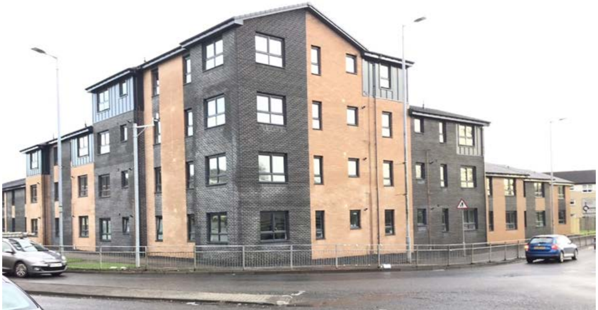
New social housing development on the former Police Station at Parkfoot Street, by Clyde Valley Housing Association (under construction)
