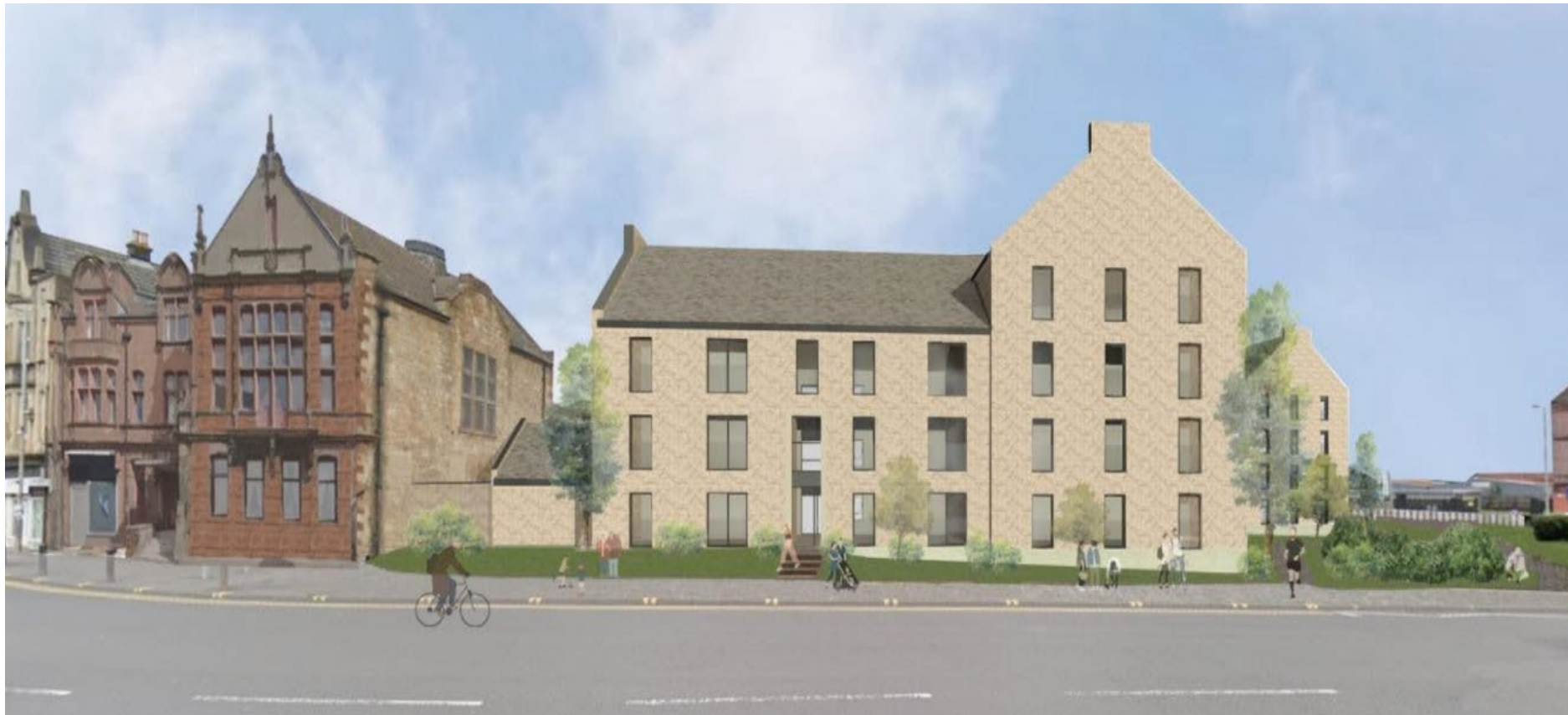
Refurbishment of the former Motherwell YMCA and New Build Flatted Blocks on Brandon Street (under construction)
