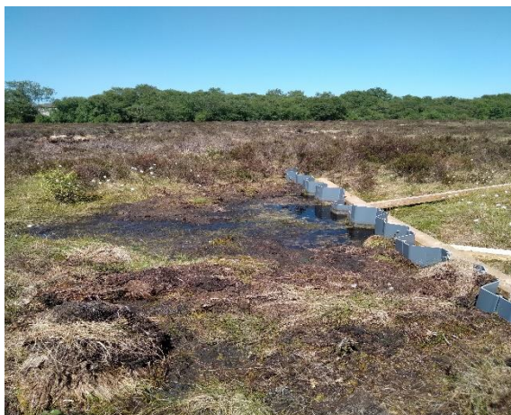
Damming works at Abronhill bog
