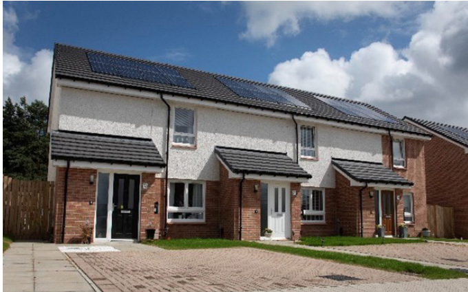
Dykehead Road, Airdrie
