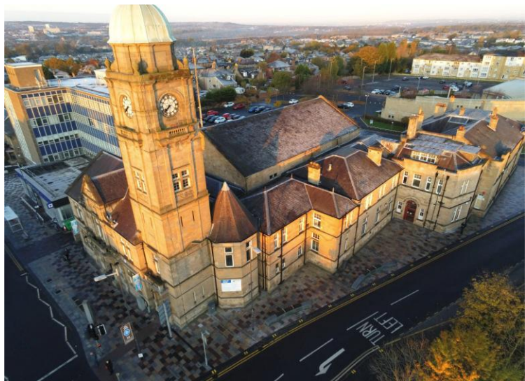
Regeneration of town centre site at Motherwell Town Hall
