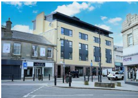
Redevelopment John Orr building, Airdrie
