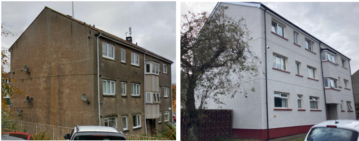
(HIBs:ABS) funded property improvements: Before and after pictures of mixed tenure blocks in Kilsyth
